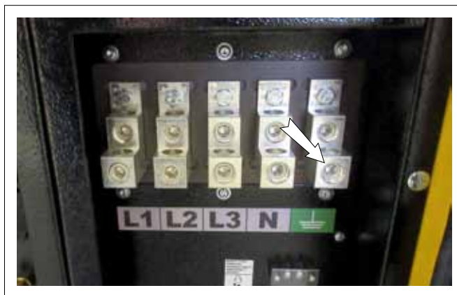
FIG. 10 GROUND TERMINAL
