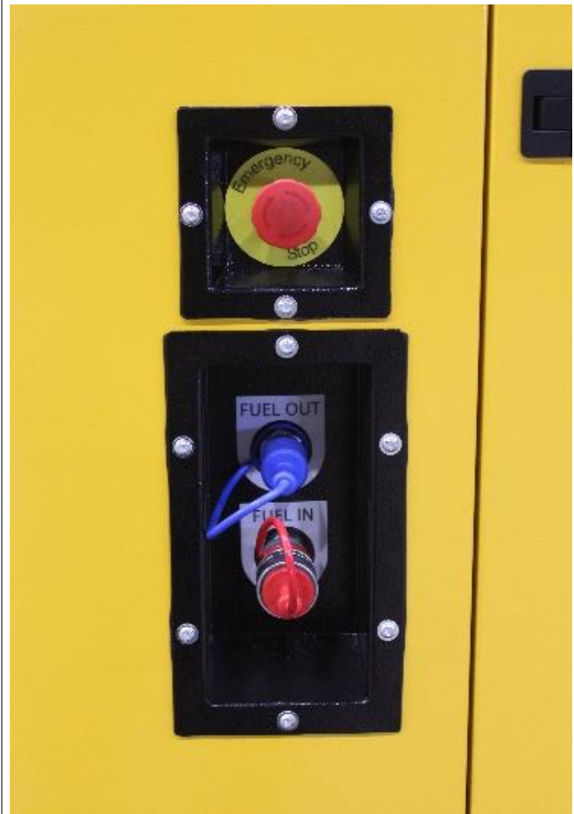
Auxiliary Tank Couplers
