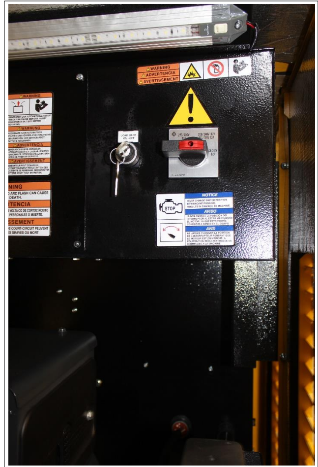
FIG. 15 LOAD BANK (TYPICAL)
