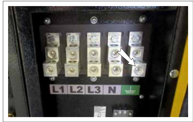
FIG. 10 GROUND TERMINAL
